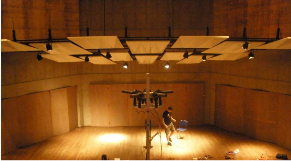
Figure 32 Adjustable height acoustic clouds for early reflection control and scattering. This photograph shows the stage in the University of Victoria's Phillip T. Young Recital Hall. The 5 channel surround sound microphone array in the foreground was used for impulse response measurements in the hall.
